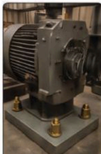
MACHINE & EQUIPMENT FIXING
