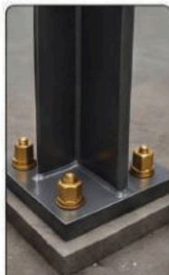
COLUMN BASE FIXING
