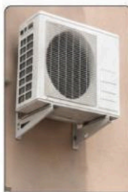
HVAC & DUCT INSTALLATIONS
